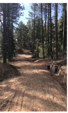
Spring roadwork also included redefining of ditches, grading, and fixing potholes throughout the neighborhood. We also improved drainage with the installation of culverts in several locations.
